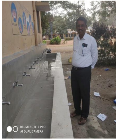
Hand wash platform
